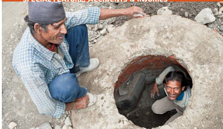
Workers repairing sewer in Manali, northern India
